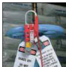
Lockout gate valves
