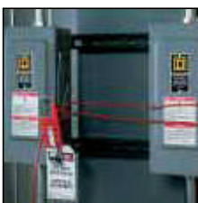
Lockout single or multiple electrical disconnects
